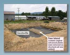
The site was excavated 60 cm deep and geotextile was placed at the bottom.
