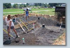
The StaLite mixture was applied to the site and then overflow drainage pipes were installed 15 cm below the soil surface (35 cm structural soil reservoir). The mixture has 34% porosity and can hold ~4.5 inches of rain.
